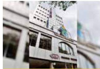
Yayasan Sarawak Building, Jalan Masjid, Kuching
