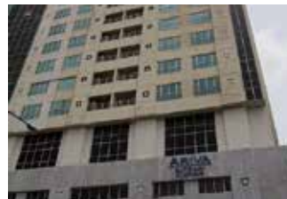
Ariva Gateway, Jalan Bukit Mata Kuching
