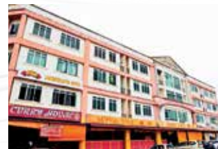
Demak Laut Commercial Centre, Kuching
